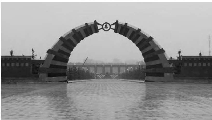
Figure 12. Federal Military Memorial Cemetery: bell arch and Kremlin wall-shaped columbarium. Behind it, the presidential avenue of the burial zone and the Pietà, Eternal Flame, and amphitheater. © Mischa Gabowitsch.
